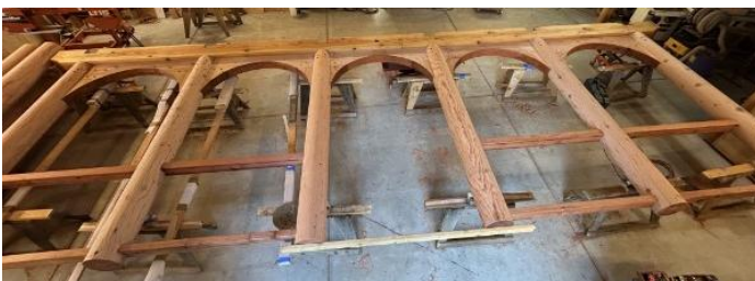
Preview of pavilion beams under construction off-site
